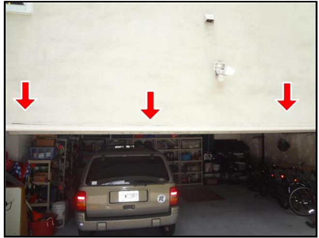
1.1 Item 2(Picture) Evidence of deflection and sagging
