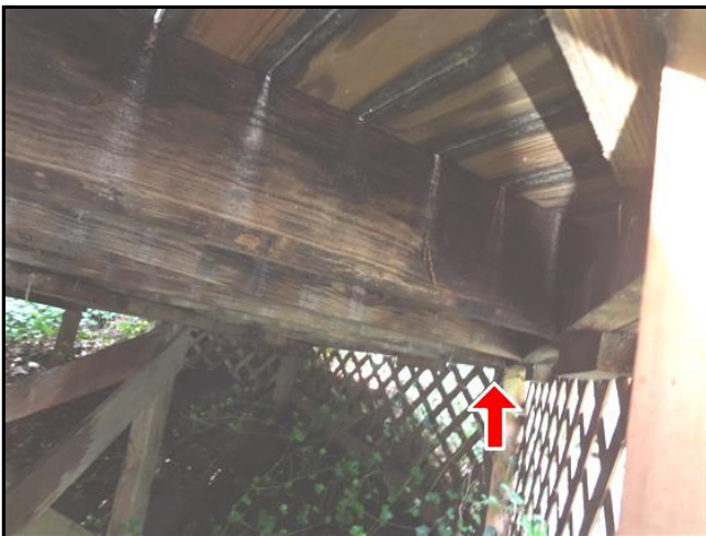
2.4 Item 13(Picture) Improper support
