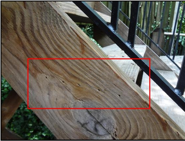
2.4 Item 23(Picture) Improper fasteners for stair string
