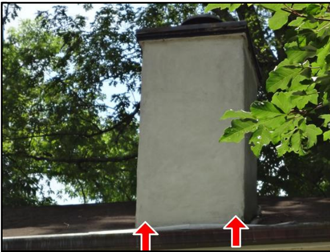
3.1 Item 3(Picture) Proper flashing needed
