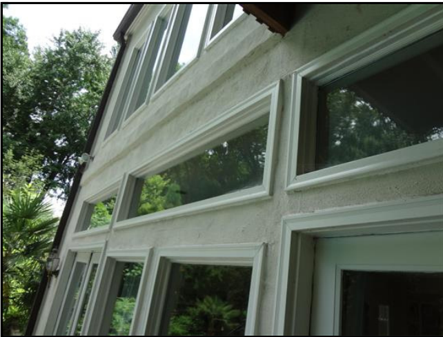
2.1 Item 5(Picture) Recommend installing drip cap flashing
