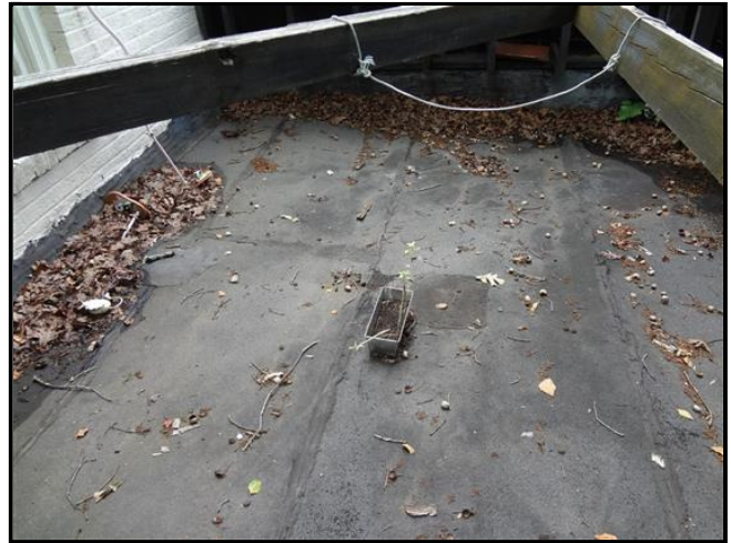
3.0 Item 2(Picture) Aged flat roof material
