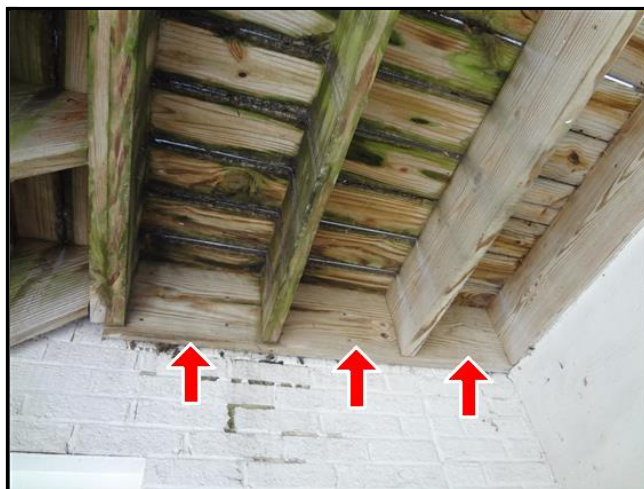
2.4 Item 10(Picture) Ledger board not properly secured
