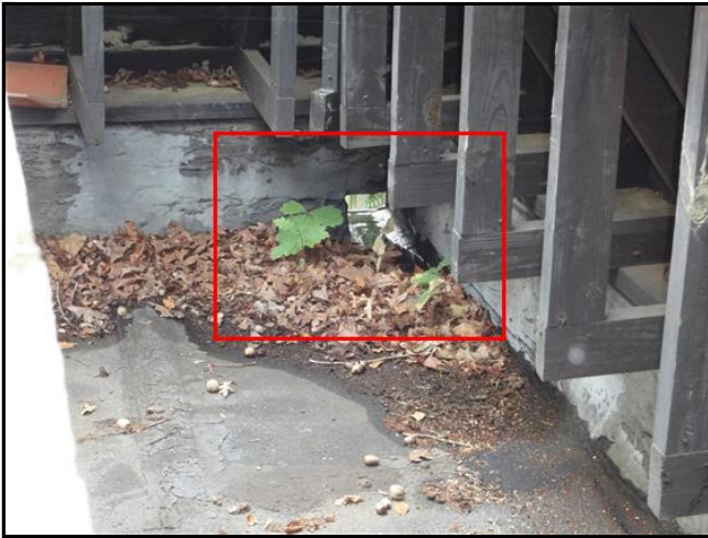
3.0 Item 1(Picture) Poor drainage design and debris clogging it
