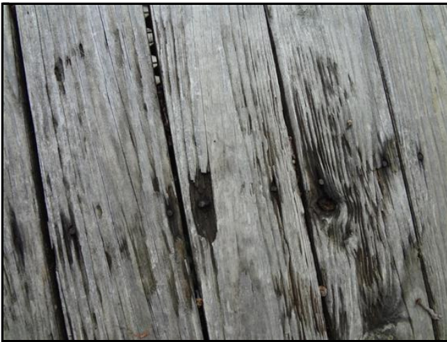
2.4 Item 25(Picture) Example of aged/deteriorated decking
