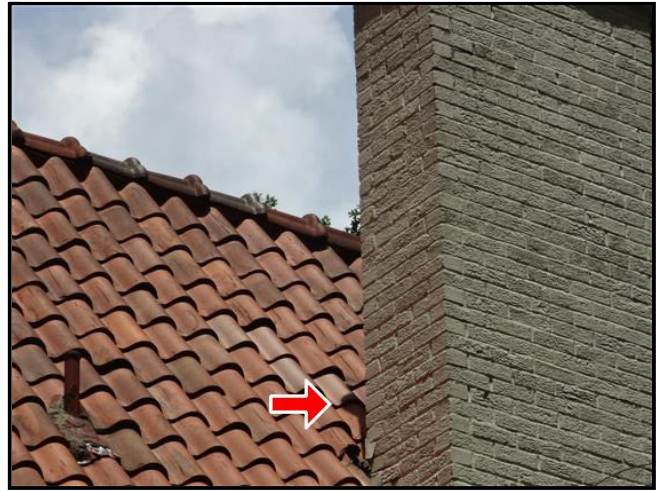
3.1 Item 2(Picture) Proper flashing needed at chimney
